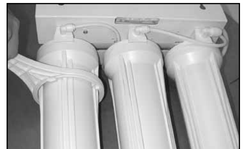
Figure 11 - Using sump wrench to change filter cartridges
